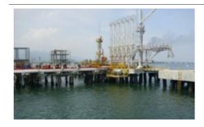
Concept and Basic Engineering for the design of a coke loading pier and a heavy unloading pier as part of the expansion project of the El Palito refinery.
