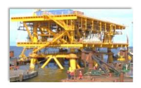
Engineering assistance for Float – Over installation of the top side of the off shore wellhead platform Corocoro
